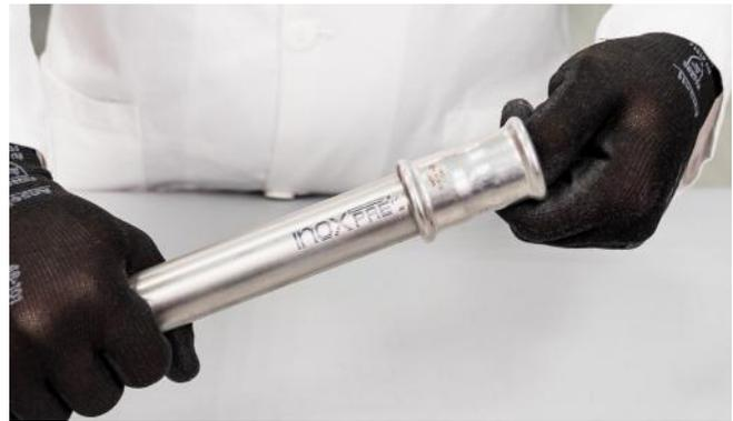
Inserting the pipe into the press fitting
