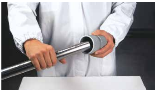
Deburring of the pipe
