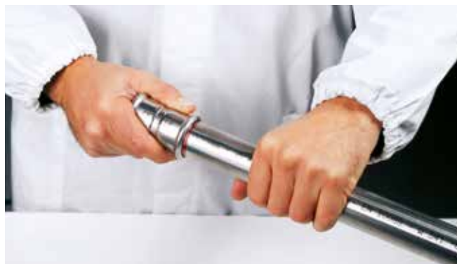
Inserting the pipe into the press fitting
