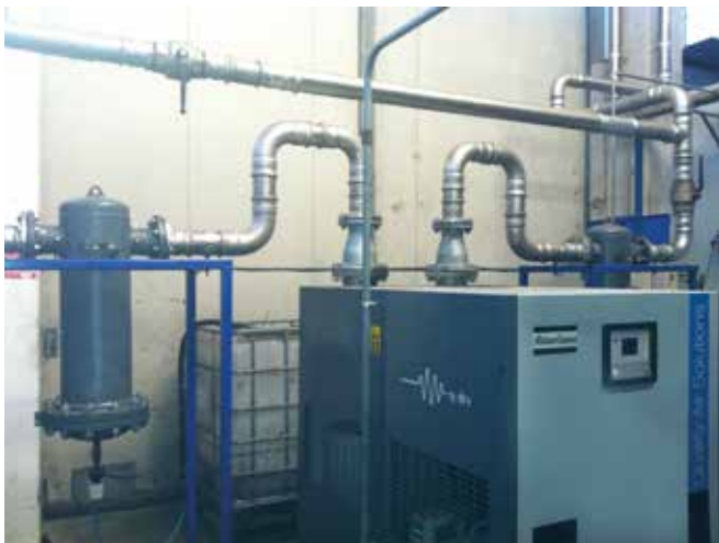
Filters with dryer
