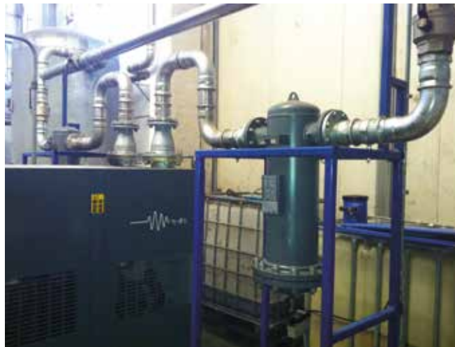
Filters with dryer
