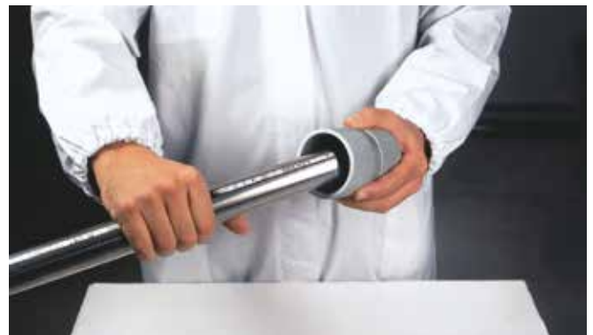
Deburring of the pipe
