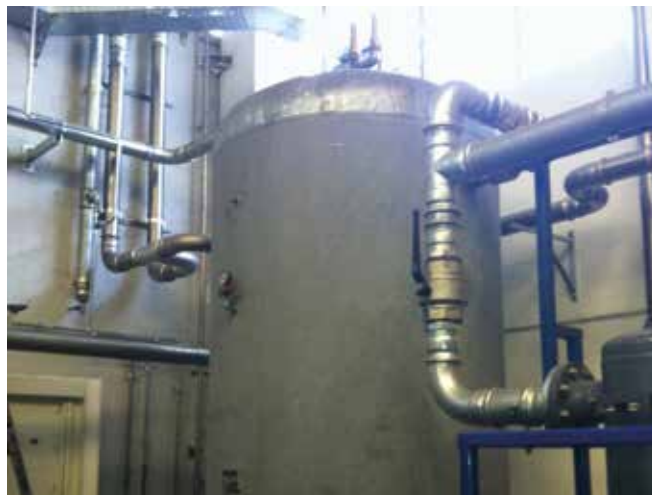
Compressed air tank
