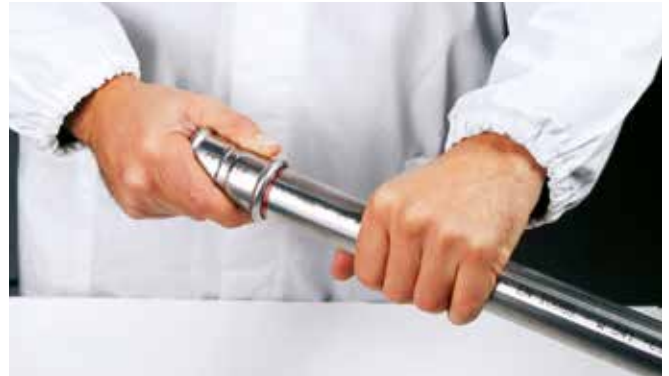
Inserting the pipe into the press fitting
