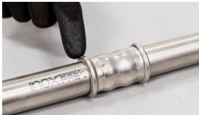
Figure 12 - Checking the press connection
