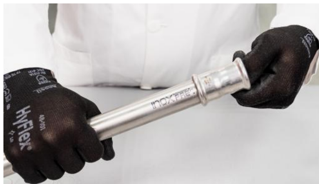
Figure 10 - Inserting pipe into the press fitting
