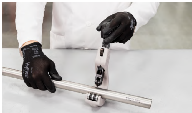
Figure 5 - Cutting the pipe to length
