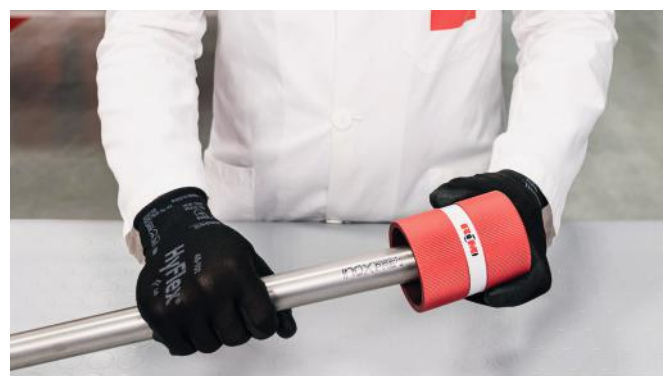
Figure 27 - Deburring the pipe
