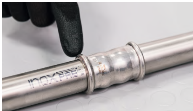
Figure 34 - Checking the press connection
