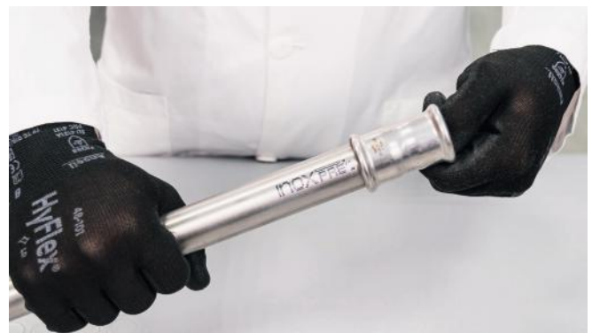
Figure 32 – Inserting pipe into the press fitting
