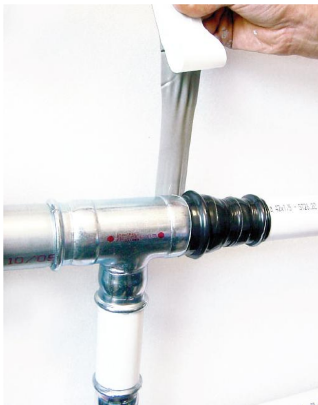
Figure 39 – Protection of the connectors with butanol adhesive tape
