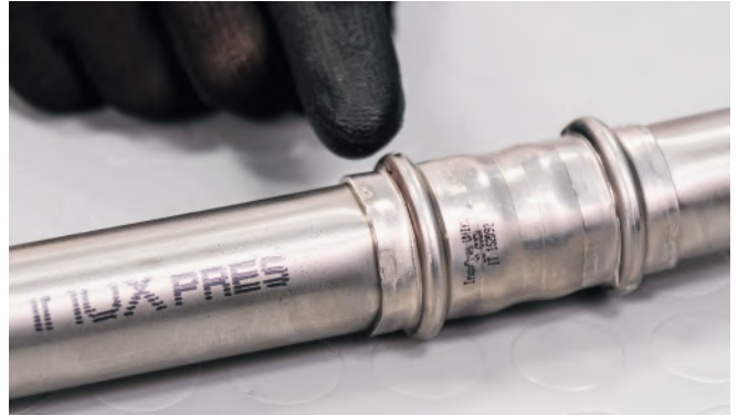
Figure 27 – Checking the press connection
