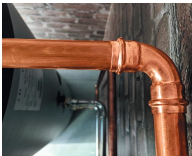
Figure 17 - aesPRES UNIKO - Heating installation
