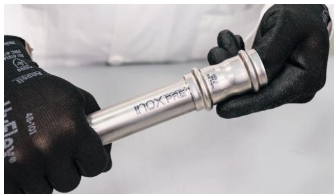
Figure 25 – Inserting pipe into the press fitting
