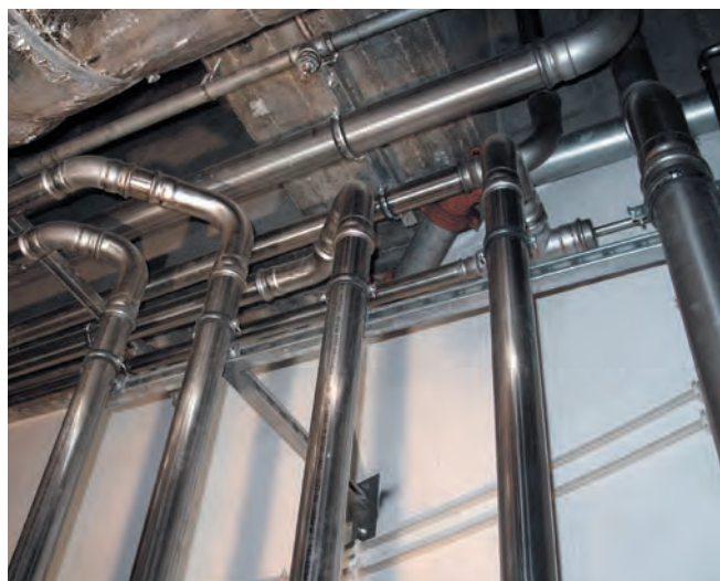
Figure 22 - inoxPRES - Example of Installation
