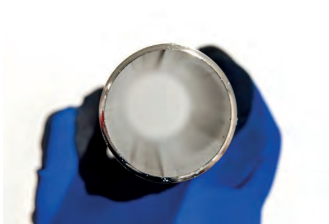
Figure 40 – Example of an Unobstructed Pipe
