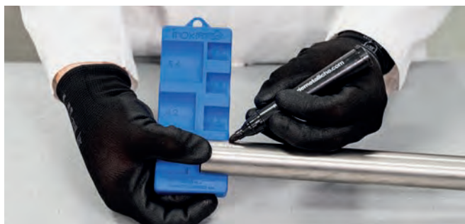
Figure 35 – Insertion Depth Marking Using a Marking Gauge Ø 15 mm – Ø 54 mm
