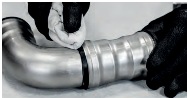
Figure 78 - Removal of Excess Lubricant
