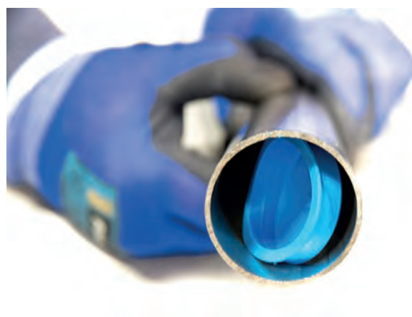
Figure 41 – Example of an Obstructed Pipe
