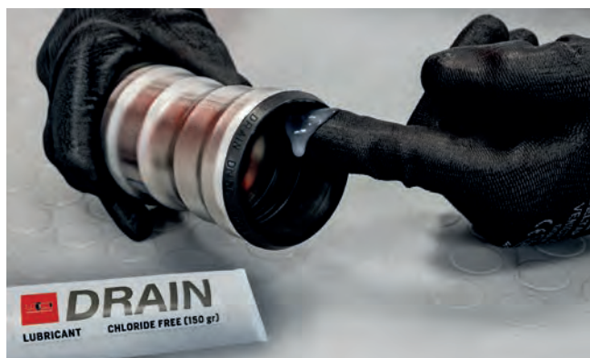
Figure 76 – Lubricating the Gasket
