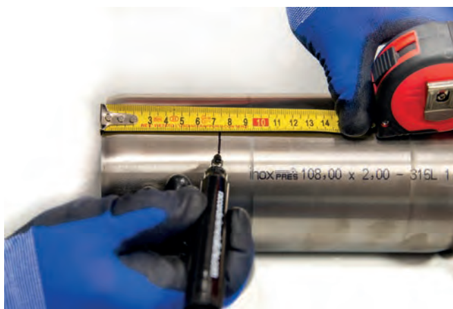
Figure 33 – Insertion Depth Marking Using a Measuring Tape
