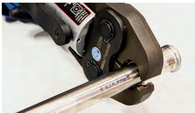
Figure 42 – Pressing the Fitting
