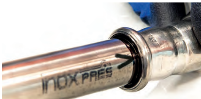
Figure 37 – Example of Incorrect Marking
