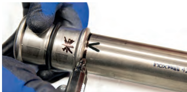
Figure 36 – Insertion Depth Marking Using a Reference Fitting
