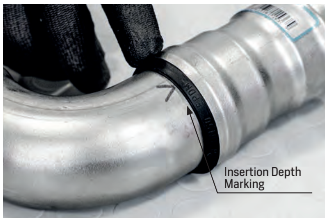
Figure 79 - Verification of Complete Pipe Insertion into the Socket
