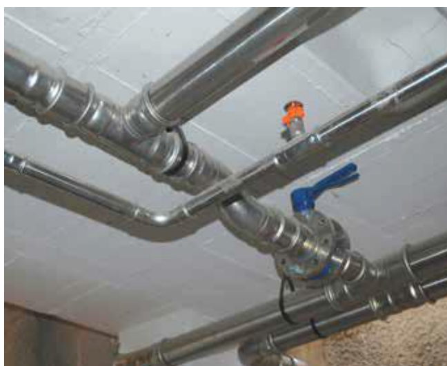
Figure 19 - inoxPRES – Sprinkler system in warehouses
