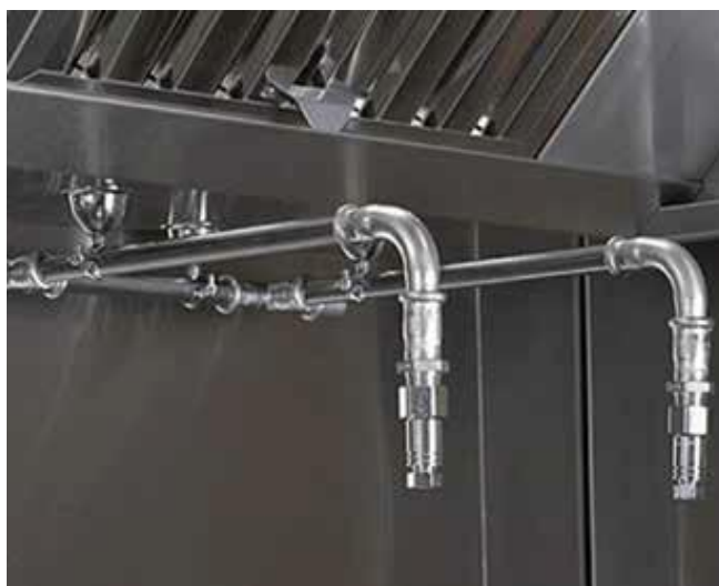
Figure 20 - inoxPRES – Sprinkler system in industrial kitchen
