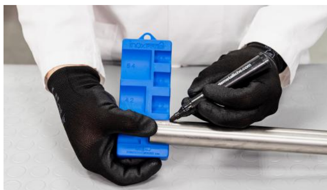
Marking the insertion depth
