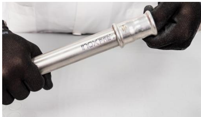
Inserting the pipe into the press fitting
