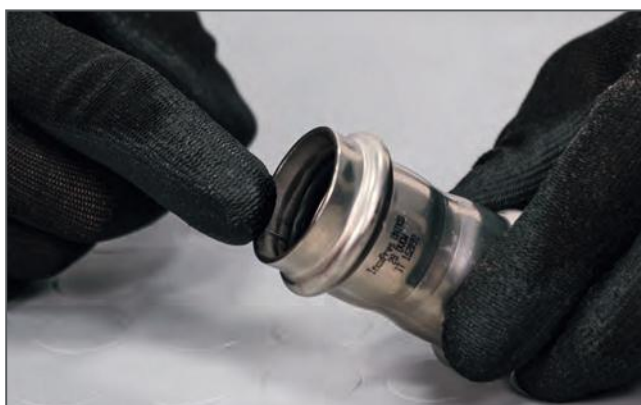
Controllo O-ring / Checking the sealing ring
